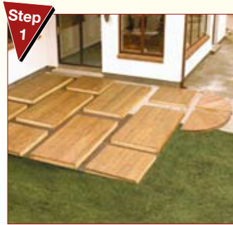
Step 1 Modular Layout Plan your deck layout in a brickwork pattern using the Vermont panels
