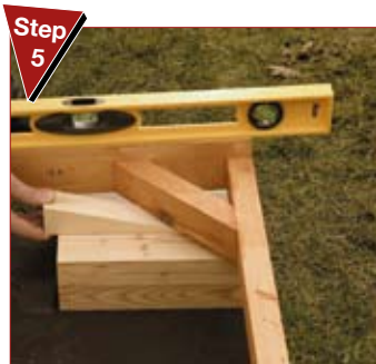
Step 5 Levelling the frame Use the easy levelling Vermont Block & Wedge system
