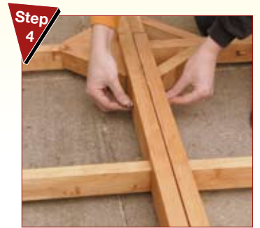
Step 4 Bolting of subframe Bolt subframe panels together
